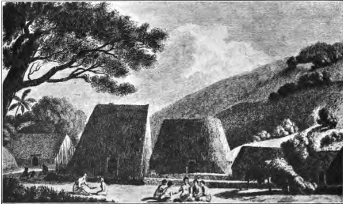
FIG. 90. ELLIS' VIEW OF HOUSES AT KEALAKEAKUA.
